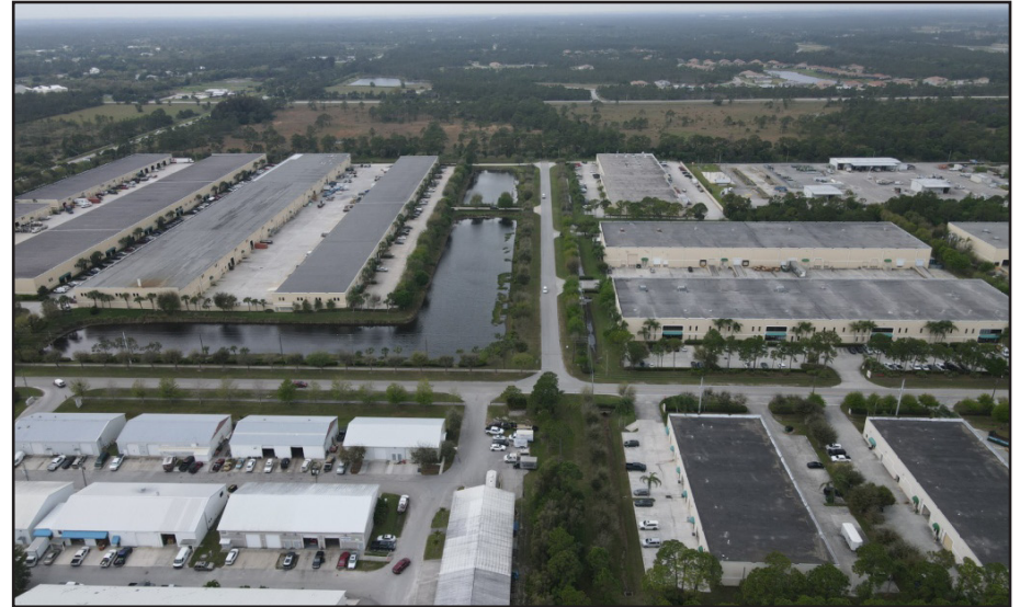
The Sands Commerce Park anchors Palm City's industrial, warehousing and logistics industries
