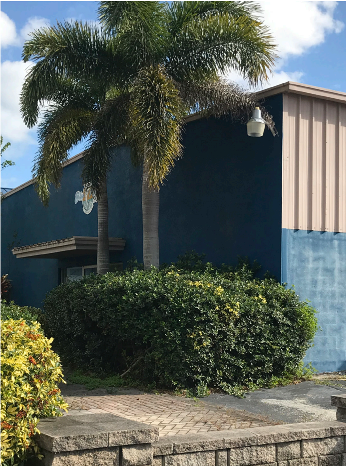
A building on the City Parcels across the street from the Civic Hub
