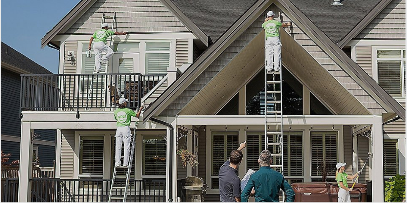
Image: Home exterior paint repair. (Source: Make Architecture Happen)
