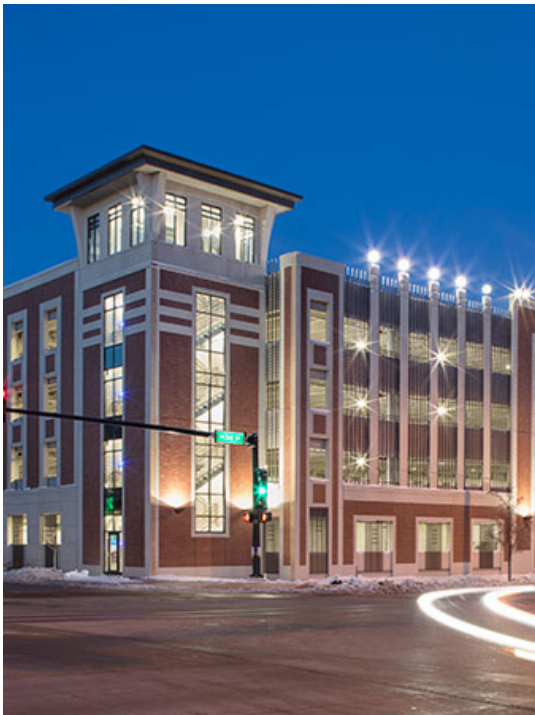
Image: An example of a centralized parking structure. (Source: Walsh Group)
