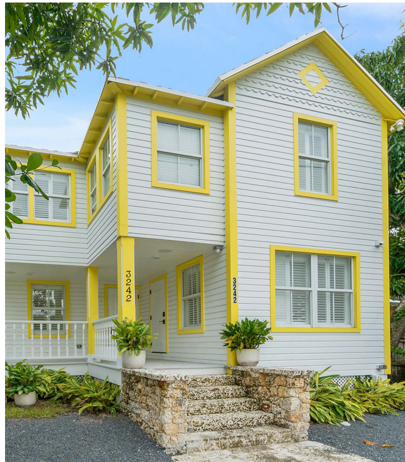
Image: E.W.F Stirrup built his house in 1897 out of Dade County Pine cut from the site and milled at the Munroe sawmill. (Source: stirrphouse.com.)
