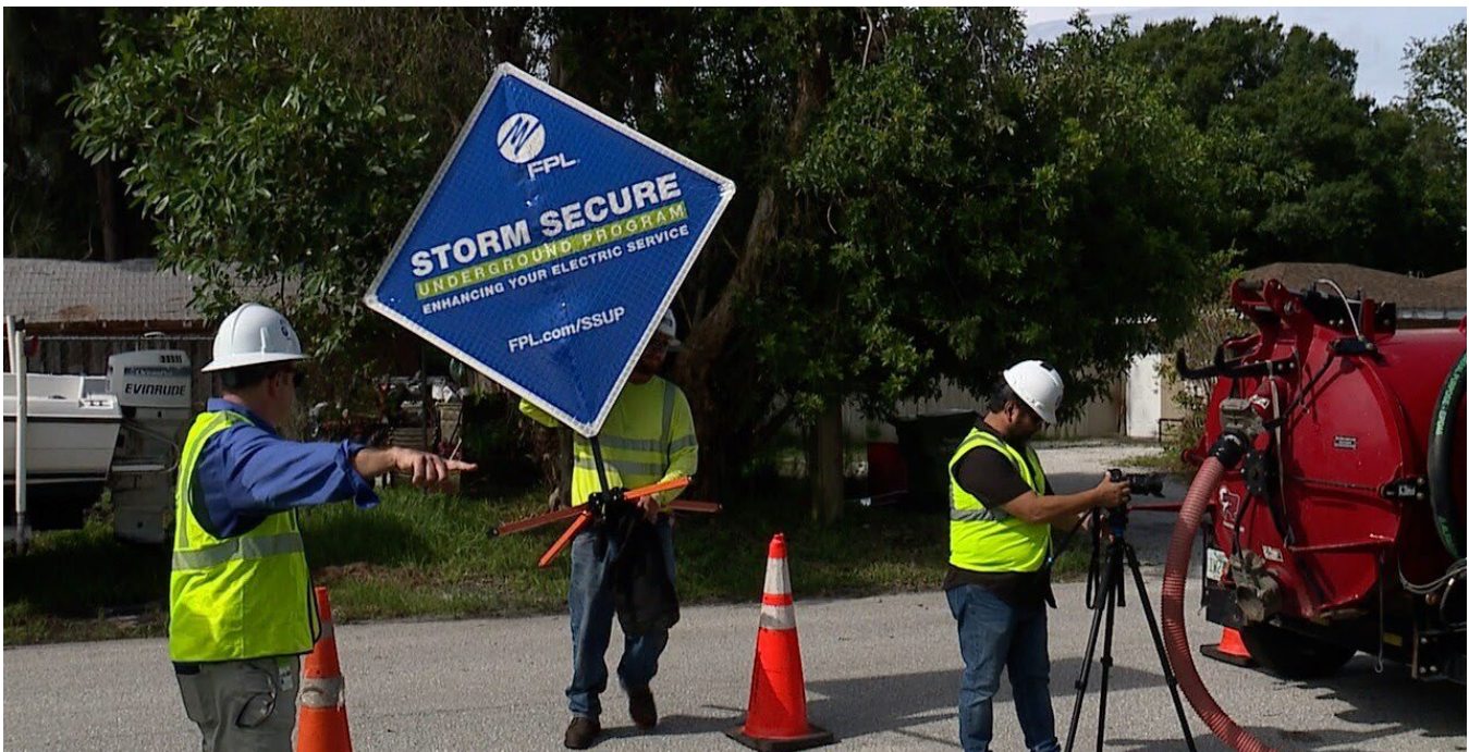
Photo: FPL Installing More Underground Power Lines
